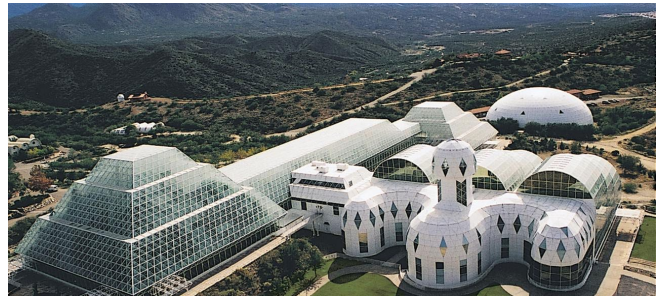
Figure 2. Biosphere 2 located in Southern Arizona is 3.14-acre indoor (previously sealed) facility designed to operate as a self-sufficient base housing 8 humans for 2 years. Two experiments were conducted in 1991 and 1993, leading to mixed results with self-sufficiency never being achieved [24-25].
